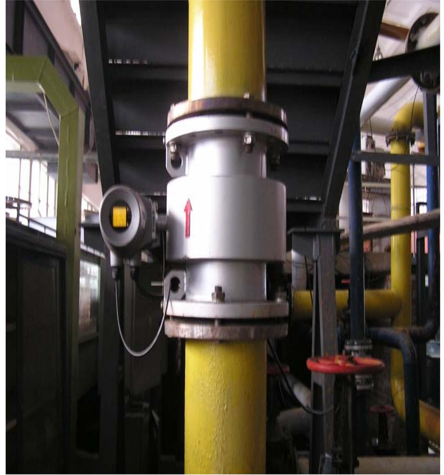
↑ The electromagnetic flow meter for the discharge and the flow velocity test
