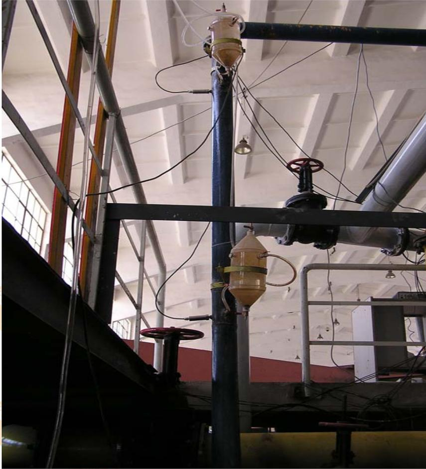
↑ the isolation pot and differential pressure sensor
